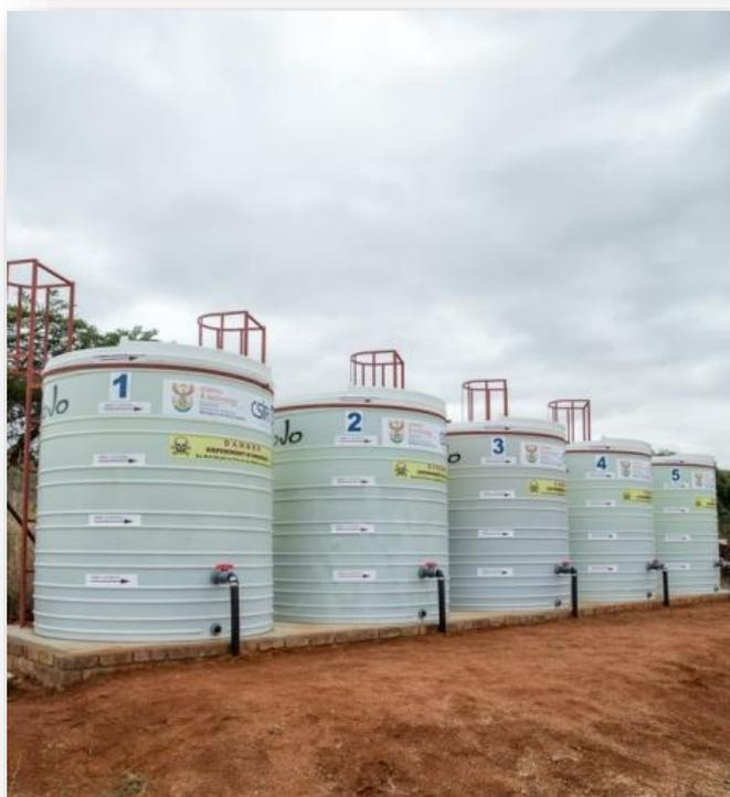
The algae bioreactors at Motetema wastewater treatment works
